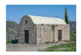
supported internally by a reinforcing arch and externally by a pair of buttresses (north and south). On the outside it was covered with a mixture of lime and concrete, a strong traditional waterproofing mixture. The church is covered inside with plaster, while there is no evidence of wall paintings, despite the fact that their presence was assumed. The chapel is a listed monument (Table B).
