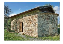
two of which at the eastern corners. It has a symmetrical arrangement and morphological elements that allow dating it to the 12th century. The vertical parts of the chapel were restored in 2012, including the reconstruction of the south-eastern part to its present form; and was covered with a simple gabled wooden roof in 2013. The chapel is a listed monument (Table B).
